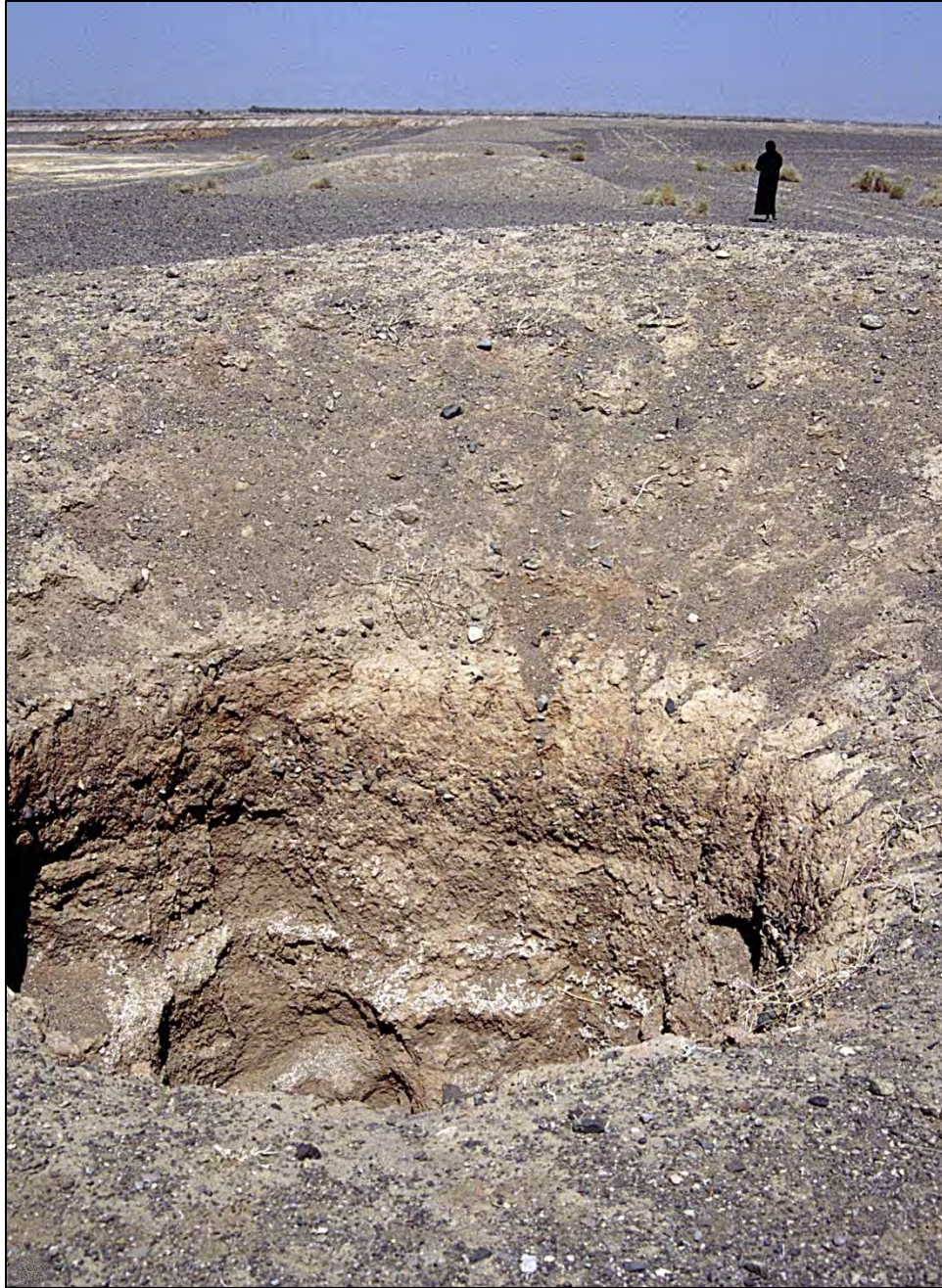
Kerman, qanat access shaft with other shafts in distance (CC BY-SA 4.0, cropped, Ziegler175).
