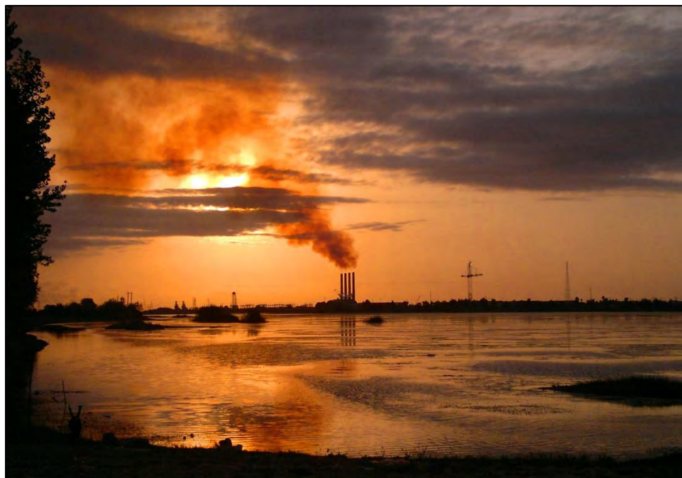
Mazandaran, Lapu Lake (view of the power plant from Lepo (in Farsi), CC BY 3.0, zs.shervin).
