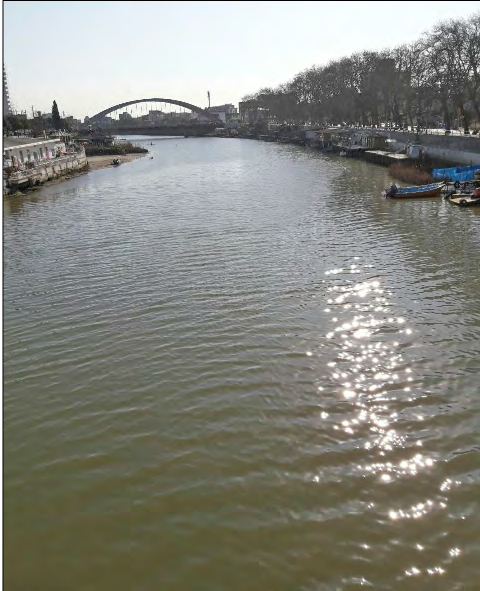
Mazandaran, Babol River (Bridge babolrood, CC BY-SA 4.0, Zpashna82).
