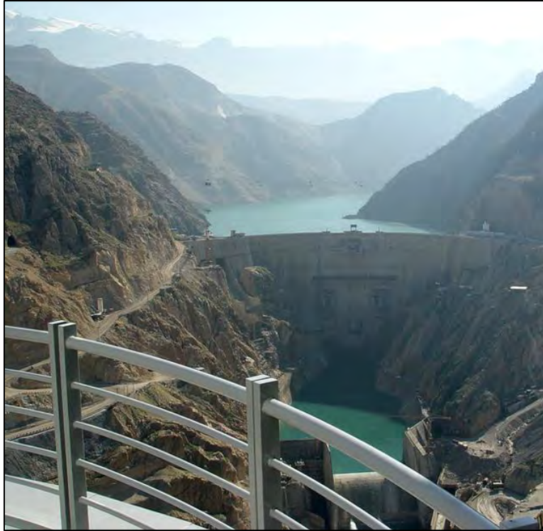
Khuzestan, Karun-3 Dam (Karun3-dam, CC BY-SA 3.0, Zereshk).
