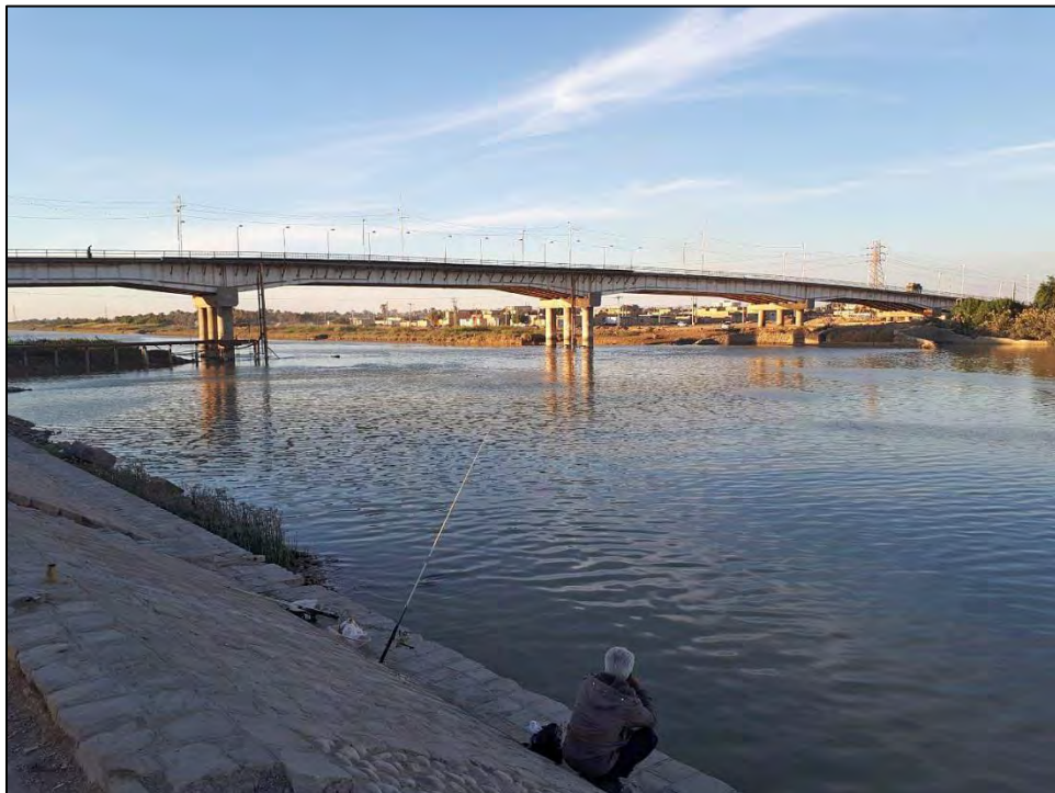
Khuzestan, Bahmanshir River, bridge at Istgah-e Haft, Abadan (Istgah e Haft Bridge Abadan Iran (1), CC BY-SA 4.0, Ahmad Darabi).
