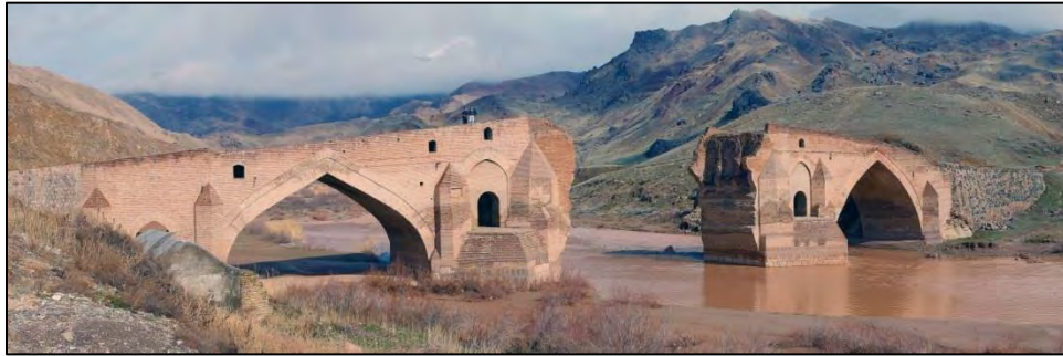
East Azarbaijan, Pol-e Dokhtar Bridge over Qezel Owzan River near Mianeh, 2013 (Kizil Hausen Bridge 2013, CC BY-SA 3.0, Sj.jamali).
