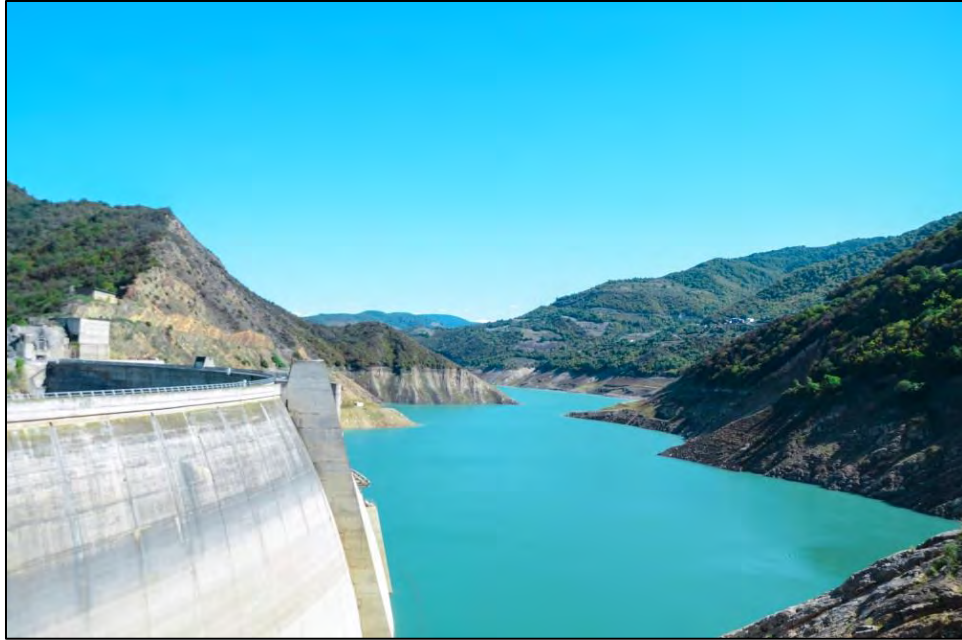
Mazandaran, Shahid Rajaei Dam (Shahid Rajayi Dam 25837656938, CC BY 2.0, #IranOpenAlbum (Negar Ghaffari)).
