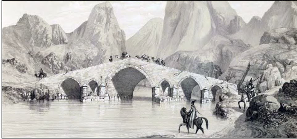
East Azarbaijan, Pol-e Dokhtar Bridge over Qezel Owzan River near Mianeh, Flandin (1840).
