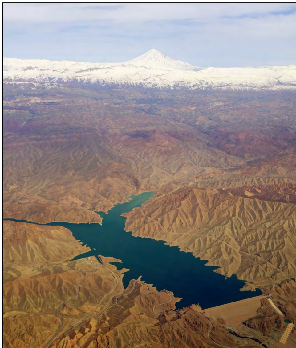
Tehran, Mamlu Dam and Mount Damavand (SadMamlooAndDamavand, cropped, CC0 1.0, Wurzelgnohm).
